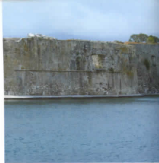
THIS FORMIDABLE ANCIENT CASTLE GUARDS THE NORTHERN APPROACHES TO THE 4NM LONG LEVKAS CANAL.
